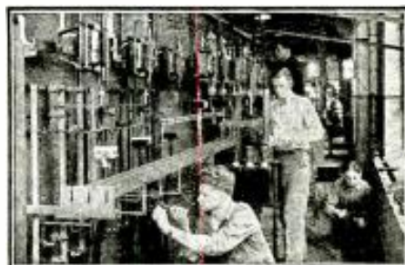
A Real Switchboard In the Coyne Shops
